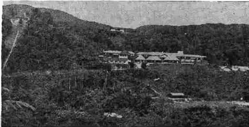
Top Left: Bukit Lowick Staff Mess. Top Centre: Hopetoun Boarding House and Staff Mess. Left to Right: In front of the School, the Assembly Hall and 3 new Classrooms. Right Front: The Pavilion and Playing Field.
